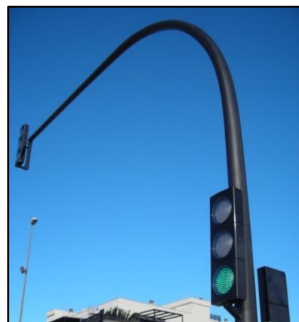
Traffic light with new casing and LEDs
