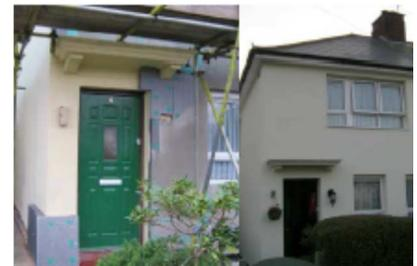
A house during and post the installation of external wall insulation.
